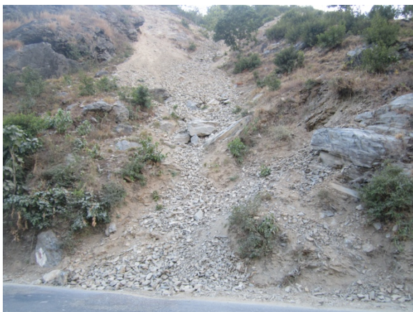
Plate11. Buinth 1 landslide along a seasonal stream
