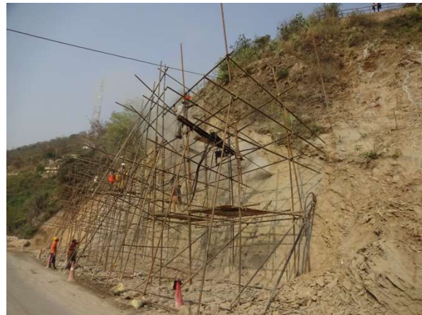
Plate 4. Rock bolting and anchoring at Devprayag 1 landslide
