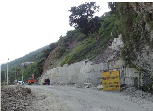
Plate 5. Retaining wall under construction at Devprayag 1 landslide
