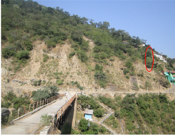
Plate 1. Bhagirathi-Bridge landslide –Local residents and Electric pole at risk
