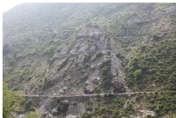
Plate 6. Devprayag 2 landslide at Pauri- Devprayag bifurcation road
