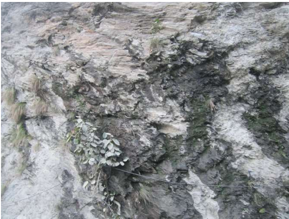
Plate 3. Seepage causing swelling in Phyllitic rocks
